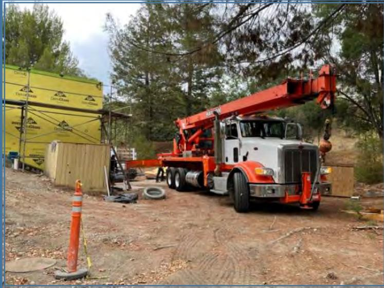
← Crane onsite used to hoist equipment onto the new kitchen roof.
