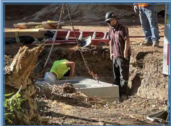
Careful installation of pre-cast concrete 750 gallon grease interceptor
